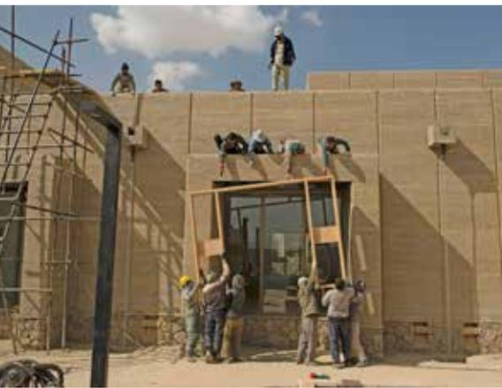
The Hospital's special low-impact, rammed-earth architecture (**above**) is designed to be not only culturally sensitive to the surrounding area, but also durable and seismic-resistant. The 400-KW solar plant (**below**) provides for the majority of the electricity supply for the Hospital.
