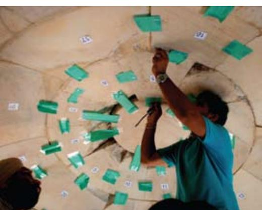
(Top) 19<sup>th</sup> century archival painting of Chausath Khamba; (Middle) A detailed architectural documentation of the structure, and (Bottom) stone-by-stone assessment of the structure showing cracks and condition of the domes prior to commencement of conservation works in 2011
