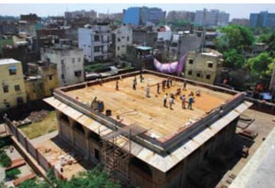
*The manner in which this complicated conservation work was undertaken bears remarkable tributes to Indian master craftsmen. (Top) Stitching and grouting of cracks in the masonry while dismantling marble blocks for repair; (Middle) Cracks on the terrace were allowing water penetration and resulting damage; (Bottom) repairs on the roof by adding a layer of lime concrete with traditional additives like Jaggery and Bael fruit pulp.*
