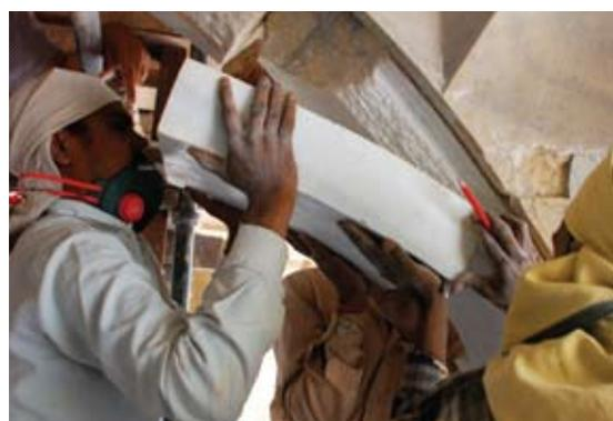
(Above) Various stages of conservation of one dome: 1. Numbering each stone; 2. Dismantling the marble blocks and repairing of cracks in the masonry; and 3. Repair of marble blocks with indents of matching stone where these had burst by master craftsmen using tools, techniques used by the original builders and 4. Re-installation of marble blocks in the original location.
