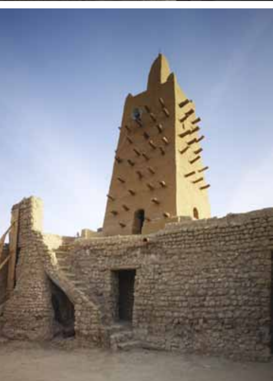
The Great Mosques of Djenné (top), Mopti (centre) and Djingereyber Mosque in Timbuktu (bottom) after restoration are all part of AKTC's Earthen Architecture Programme.
