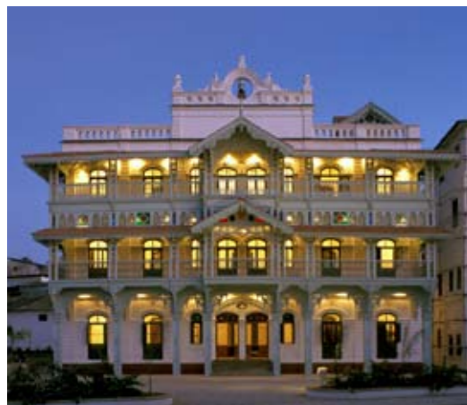
The Stone Town Cultural Centre, formerly the Old Dispensary, before and after restoration. The Centre is the future home of the Indian Ocean Maritime Museum.
