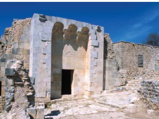
The mosque and palace of the Citadel of Salah ad-Din, both AKTC projects, were restored using materials and techniques identical to those employed by medieval craftsmen.
