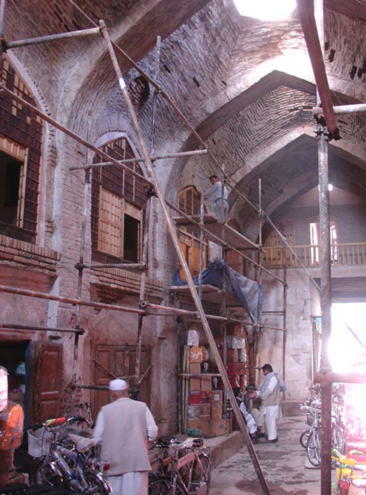
On-going rehabilitation of the interior space of the serai
