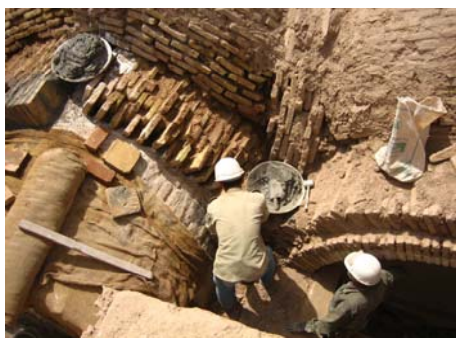
Repairs to brick masonry vaults flanking the serai
