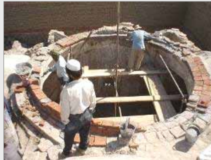
Re-building of a brick masonry dome using traditional techniques
