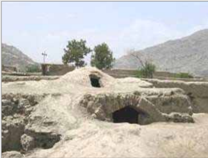
The ruined hammam prior to restoration
