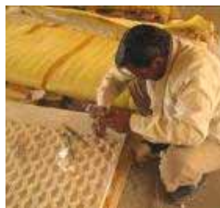
Marble waterfall being carved prior to its installation between the terraces
