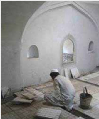
Work on the interior of the communal bathing spaces
