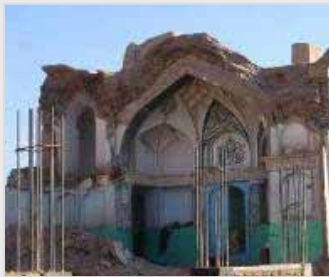
Demolition of an historic house which had been subdivided between inheritors
